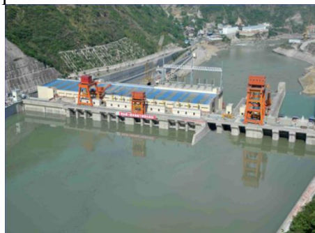
Figure 1: Power station of Zhentou-I Dam.
