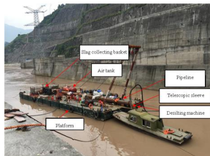
Figure 4: Pneumatic dredging system.
